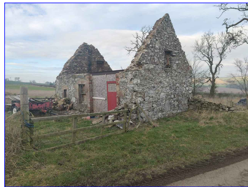
Image 10 - View of Existing Building from adjoining Highway
