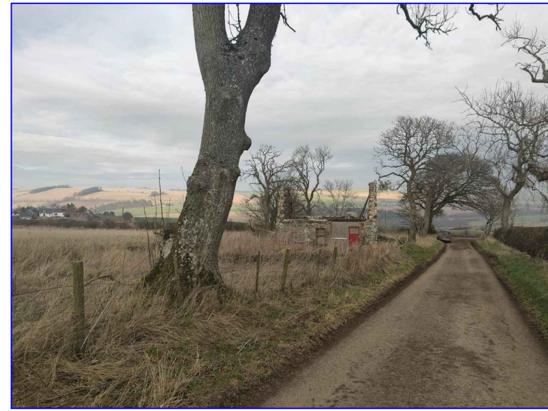
Image 02 - View of Site & Existing Building from South West Approach
