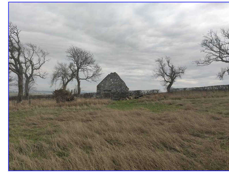
Image 09 - View of Site & Existing Building from North West Extents
