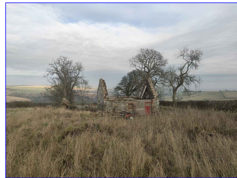
Image 11 - View of Existing Building from South West
