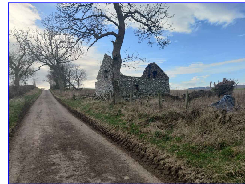
Image 13 - View of Existing Building from North East Approach
