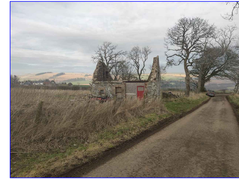
Image 05 - View of Site & Existing Building from South West Approach
